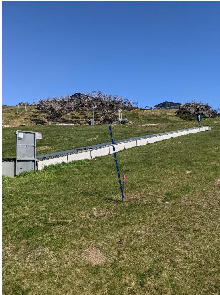
Figure 14: Alignment of new Skier Conveyor #5
